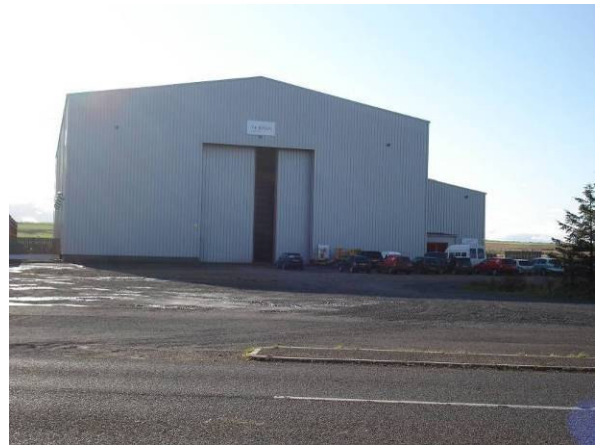
Photo 3.12 – Bower (Numax Group Facility)
