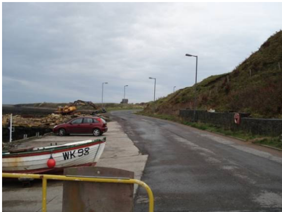
Photo 3.5 – Gills Bay, Approach Road
