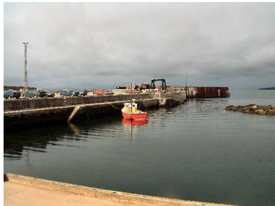
Photo 3.6 – Gills Bay, Quayside
