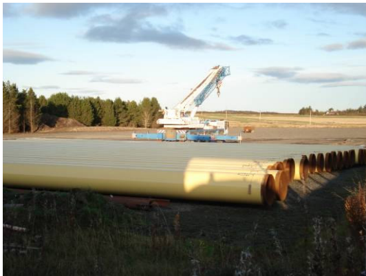
Photo 4.1 – Pipe Storage, Georgemas Junction
