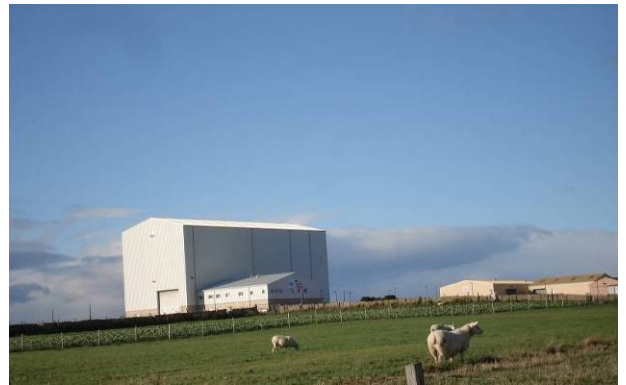
Photo 3.11 – Janetstown (JGC Engineering and Technical Services Ltd)
