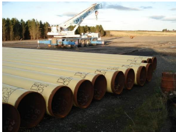
Photo 3.10 – Pipe Storage, North Side
