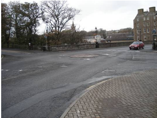
Photo 4.12 – B9159 River Street and A99 Cliff Street (From Cliff Street)
