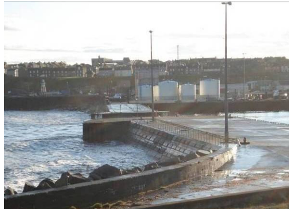
Photo 3.2 – Heavy Lift Quay, Wick
